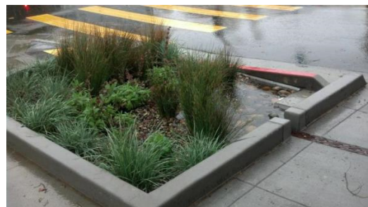
The Cesar Chavez Streetscape Improvement project included 18 rain gardens along more than a half mile of impervious street.
